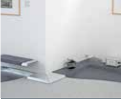
On-floor installation trunking
