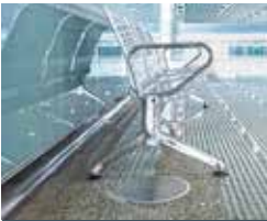
Wet-cleaned service outlets
