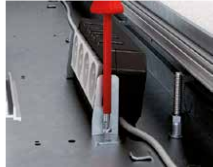
Mounting of mounting box and module support in trunking base After connection of the accessories, mount the device support on the module support or mounting box. Screw the complete unit into the trunking base.
