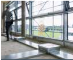
EÜK underfloor installation duct
