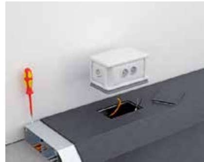
Floor covering work, mounting lid For lids with installation or set-up openings, the protective mounting lids are removed and, after application of the floor covering, the mounting openings are cut out cleanly.
