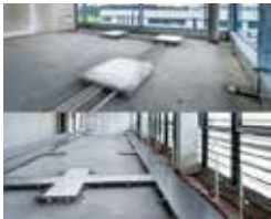
Underfloor installation duct for thin screed layers
