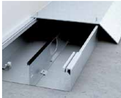
Floor covering work When laying the floor covering, ensure that it joins the trunking base. Cover the surface of the trunking lids completely with the floor covering. Pierce the floor covering on the lid fixing holes. Insert screws here and screw the lid to the trunking base.
